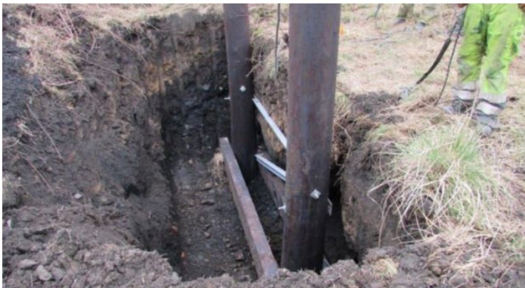
Photo 2.7: Wood pole foundations
