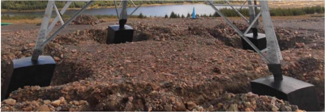
Photo 2.9: Typical Steel Lattice Tower Foundation
