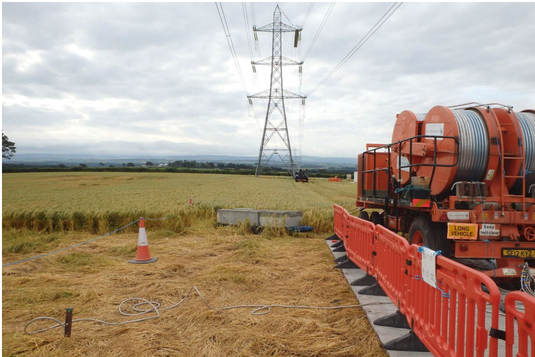
Photo 2.11: Stringing of a tower
