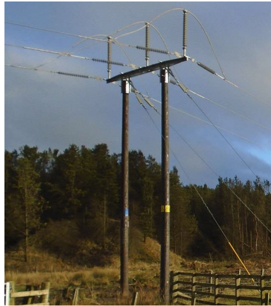
Photo 2.2: Typical H - Pole
