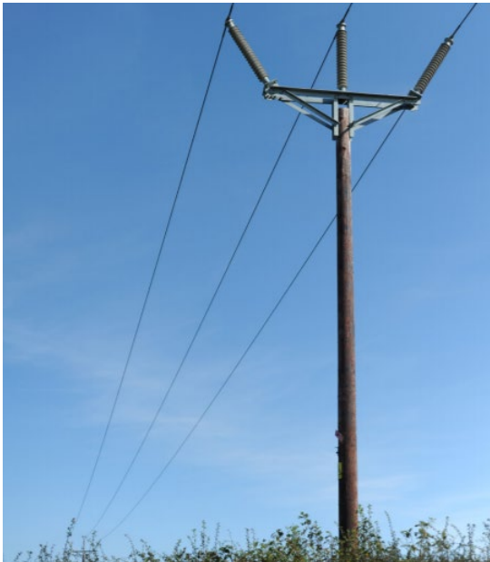
Photo 2.1: Typical Trident Wood Pole
