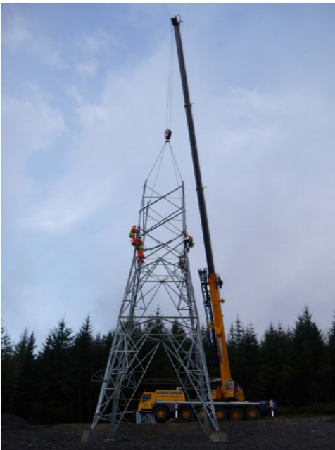
Photo 2.10: Tower under Construction
