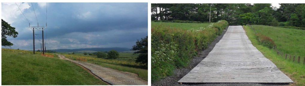
Photos 2.5 and 2.6: Temporary steel matting and timber roadway
