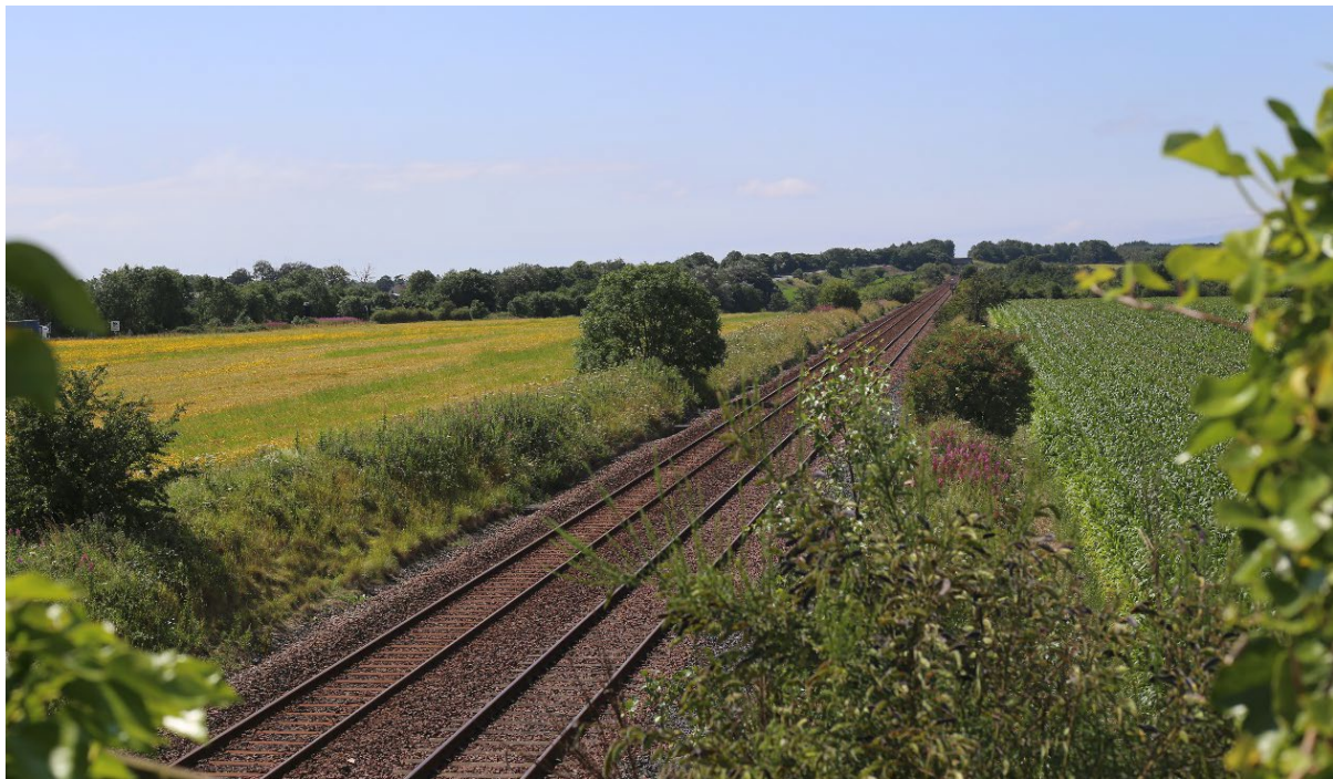
Photo: Glasgow South Western Line railway
