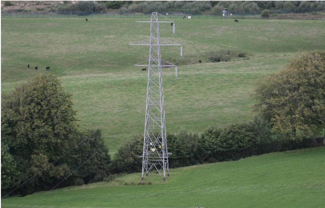
Photo 2.4: Single Circuit Steel Lattice Tower with conductors only on one side
