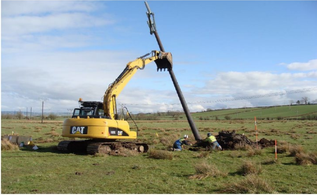
Photo 2.8: Erection of an intermediate pole
